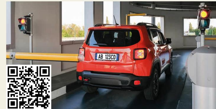
License Plate Recognition allows system operators to identify, track and analyse vehicles at entry and exit points. Automatically capture license plates in both, stop & go and moving traffic to review later or automatically open barriers or denies access removing the need of a dedicated LPR operator.
